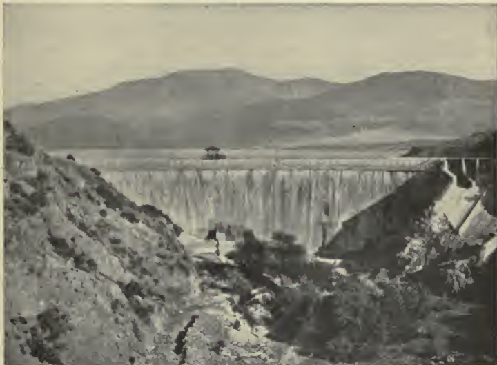
FIG. 116.—SWEETWATER RESERVOIR, NEAR SAN DIEGO, CALIFORNIA
